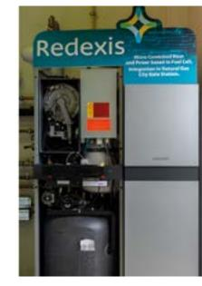
By means of a previous reformer, hydrogen is obtained from natural gas. This hydrogen reacts with oxygen in the air, producing electricity, useful heat and water.
